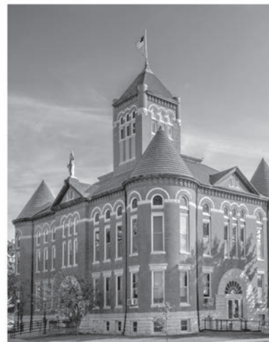
Anderson County Courthouse
